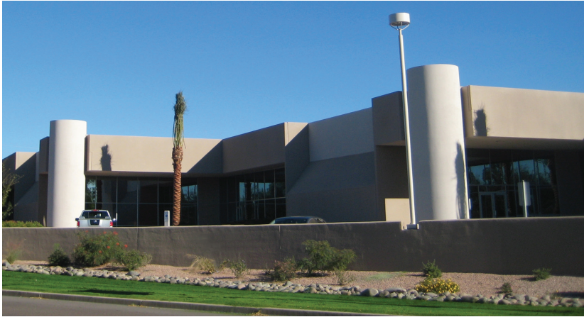
HES moved to their new LEED Silver facility in Phoenix, Arizona in the summer of 2011.
